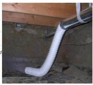
Sometimes they will terminate just beneath attic ventilators. This is a defective installation. They must terminate at the exterior and away from a door or window. Also, screens may be present at the duct termination and can accumulate lint and should be noted as improper.
